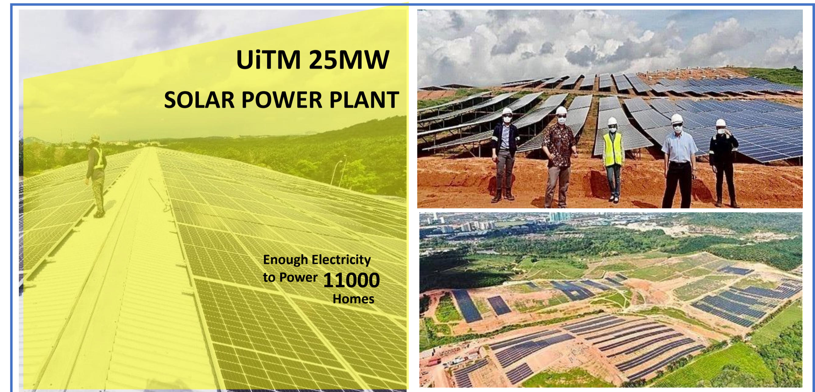
UiTM Solar Photovoltaic Plant in Pasir Gudang, Johor
