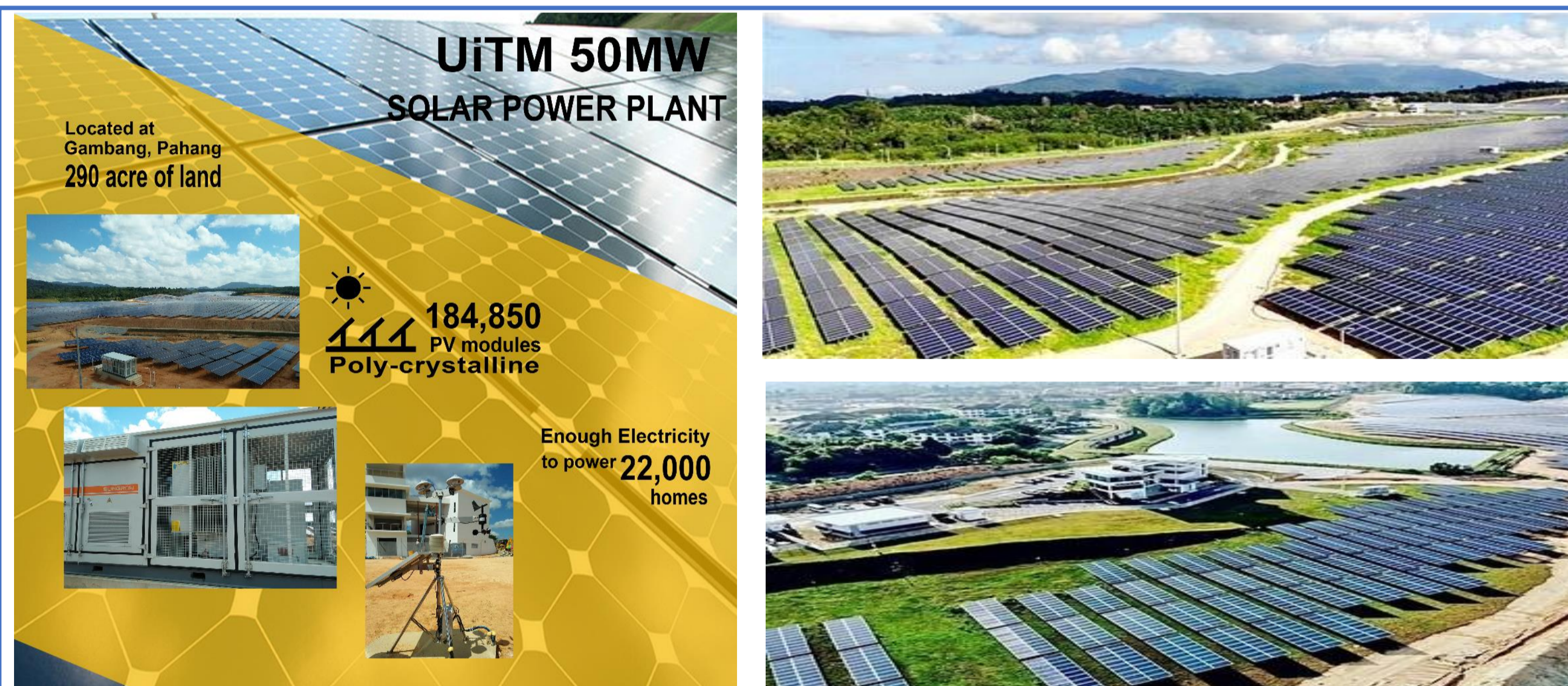
UiTM Solar Photovoltaic Plant in Gambang, Pahang
