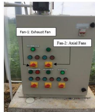
Control panel of the relays
