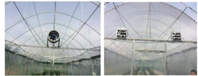
Axial fan (left) and exhaust fan (right) arrangement in the greenhouse
