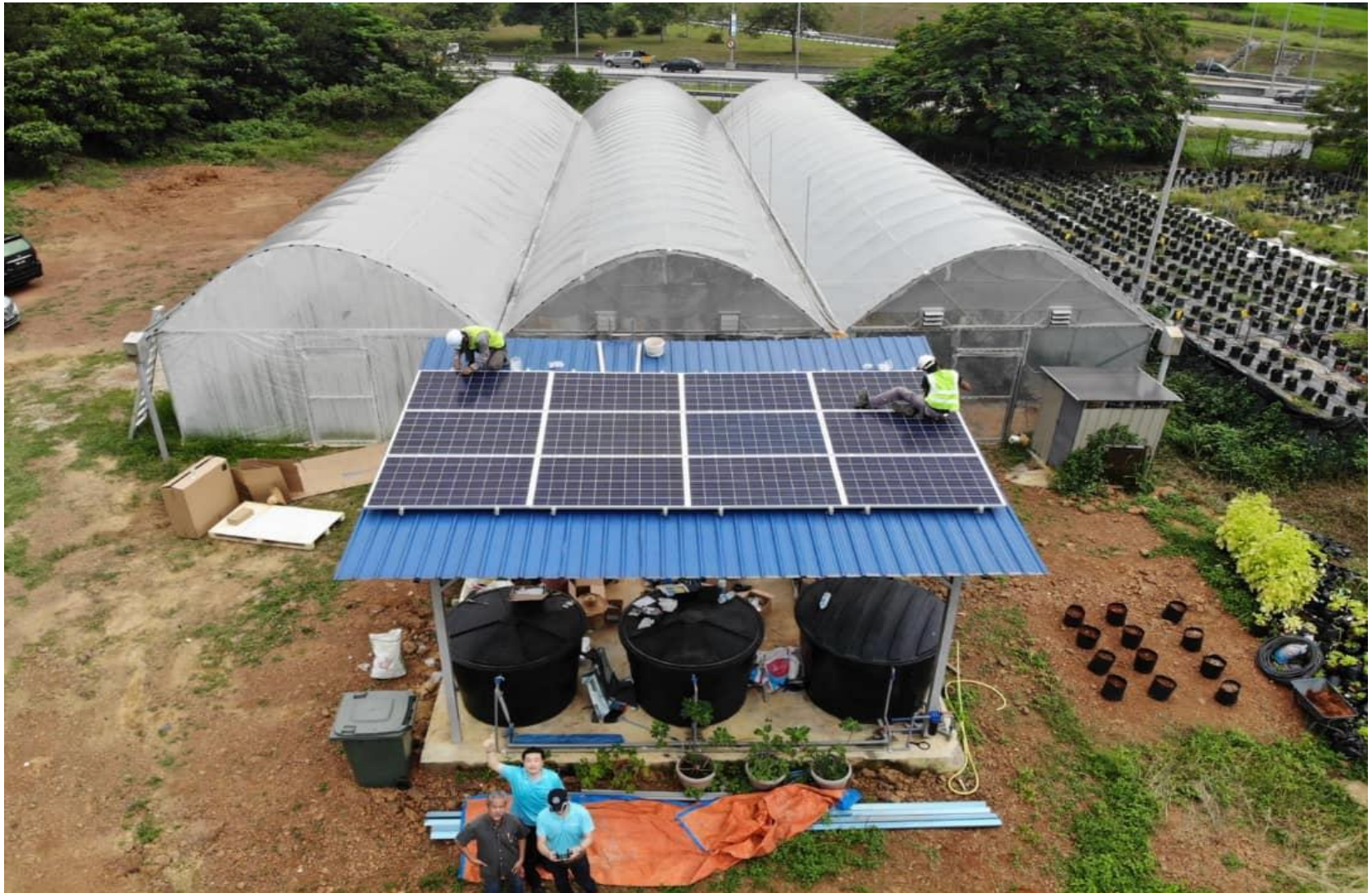
SMART GREENHOUSE SYSTEM FOR TOMATO GREENHOUSE AT UPM, SERDANG
